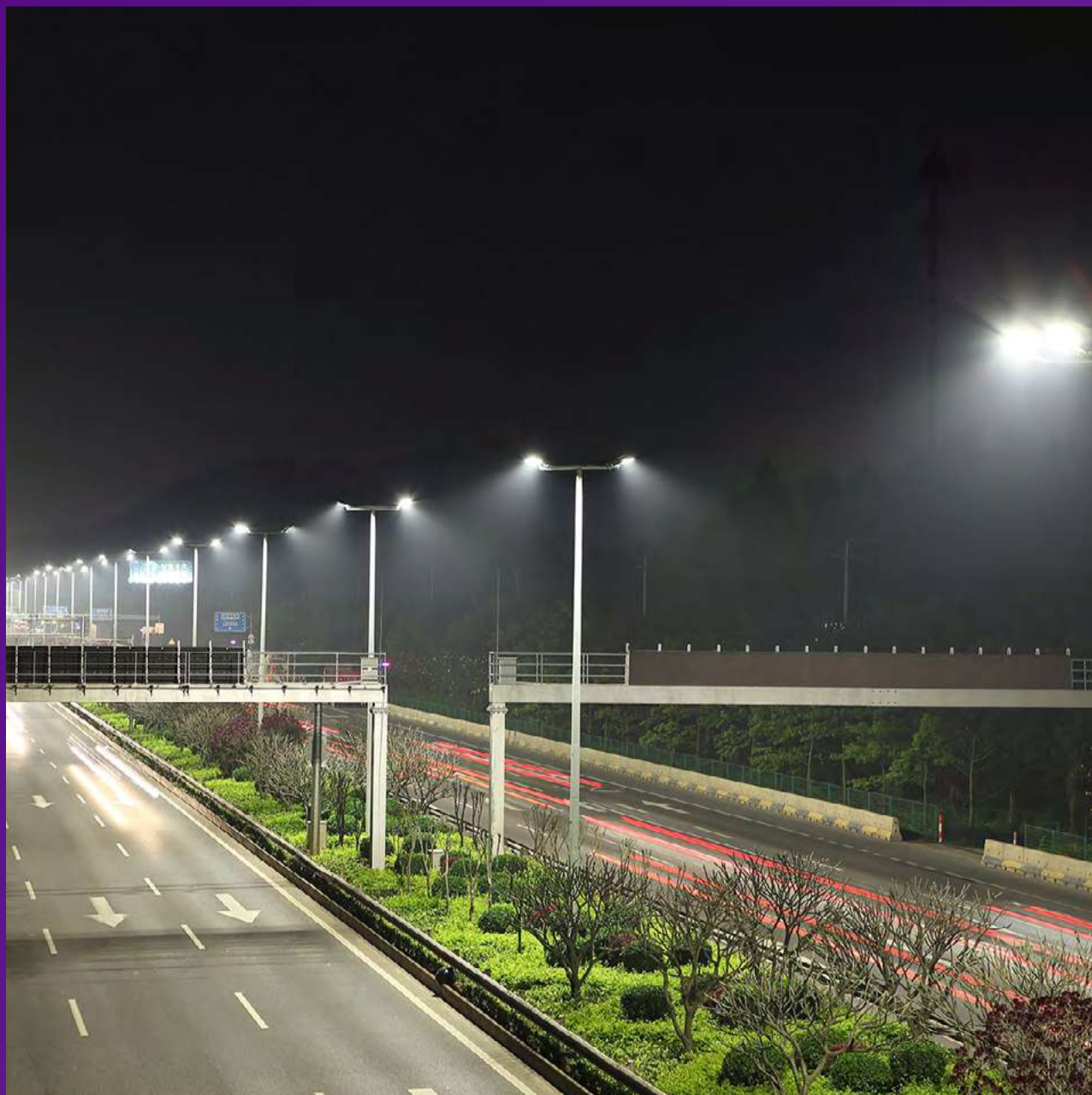
Uniform expressway lighting
