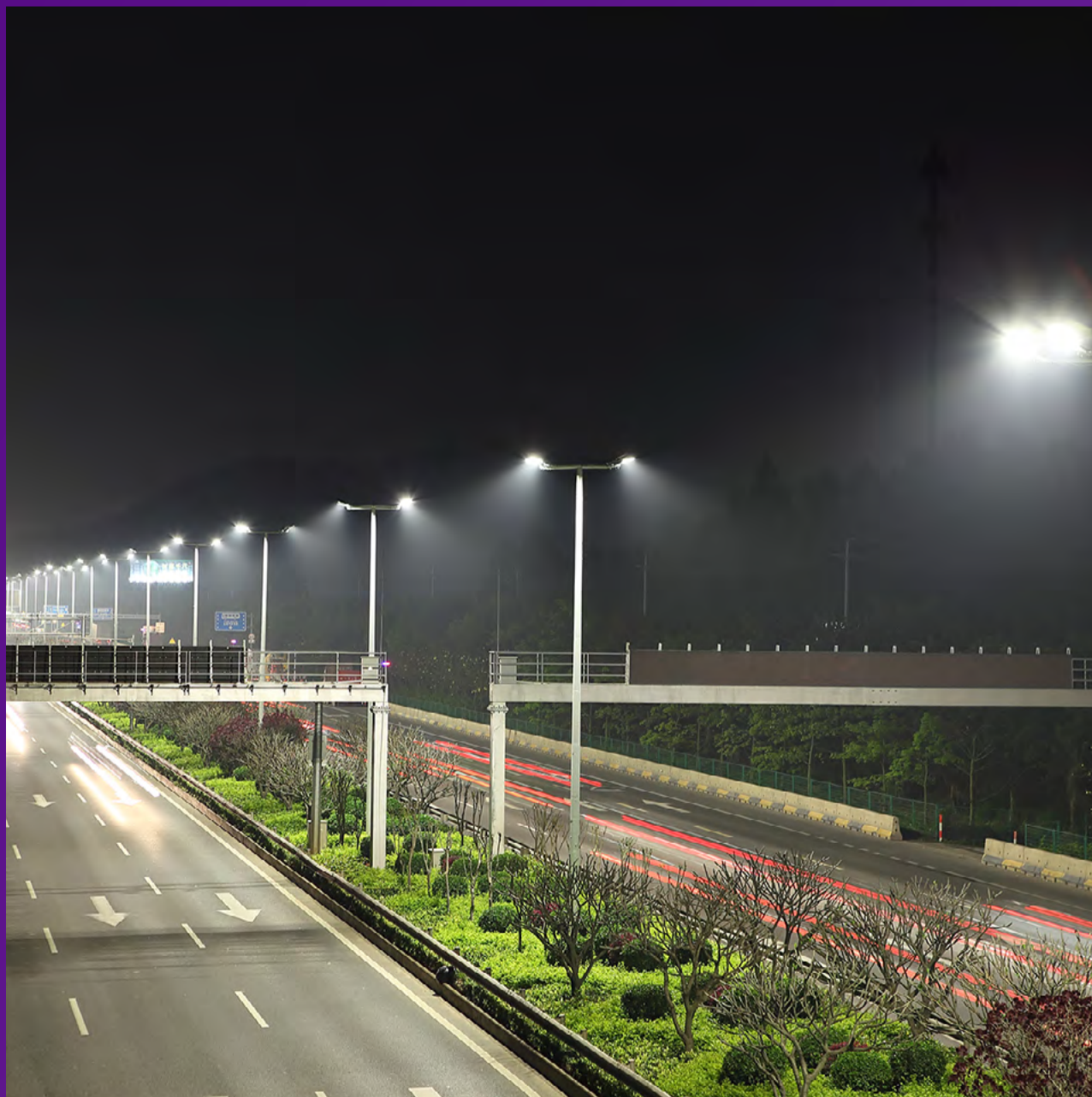
Uniform expressway lighting
